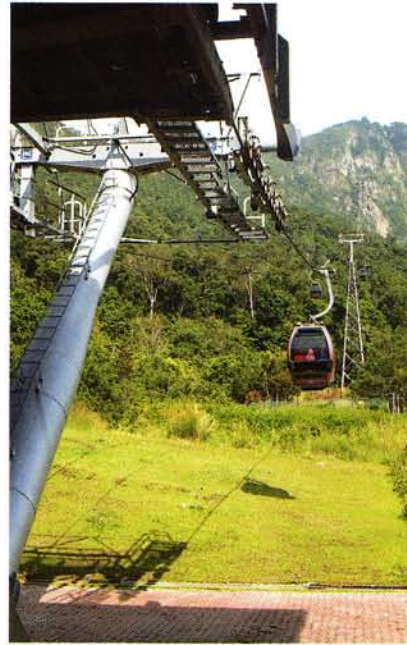
The cable-car takes you high up to a mountain lookout and suspension bridge. Both the ride and the bridge are extraordinary experiences - not to be missed!
